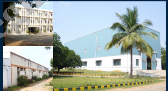
Hydraulic Cylinders & Marine Systems Plant
